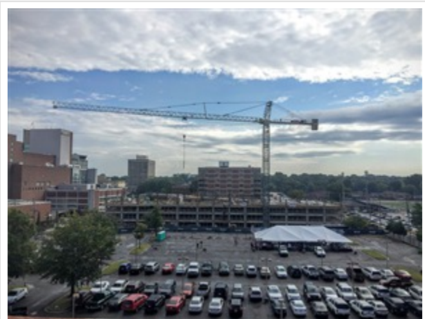
Methodist University Hospital held an official ground-breaking event Wednesday, Oct. 5, for its $280 million campus master plan at the corner of Eastmoreland Avenue and Bellevue Boulevard.
